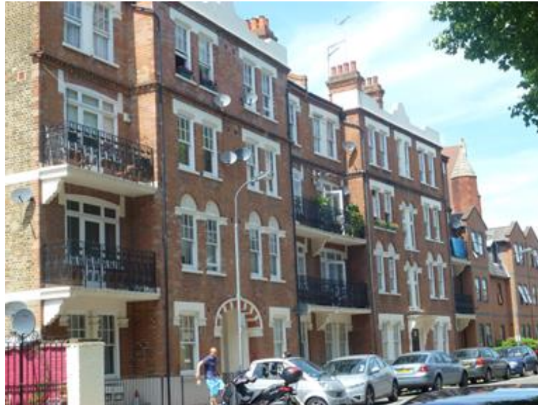
Ravenscourt Park Mansions, exuberant Dalling Road elevation unfortunately peppered with satellite dishes.
