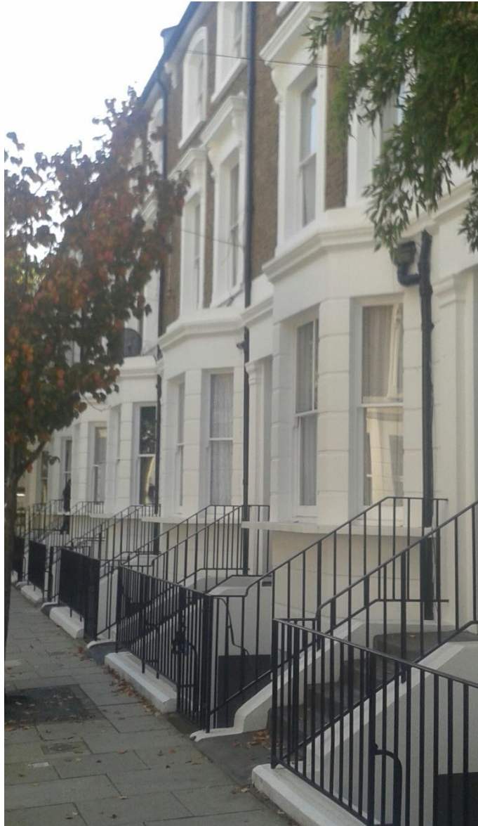
Nos. 1-13 have lost the original iron railings but fortunately the modern replacements are uniform in this group.
