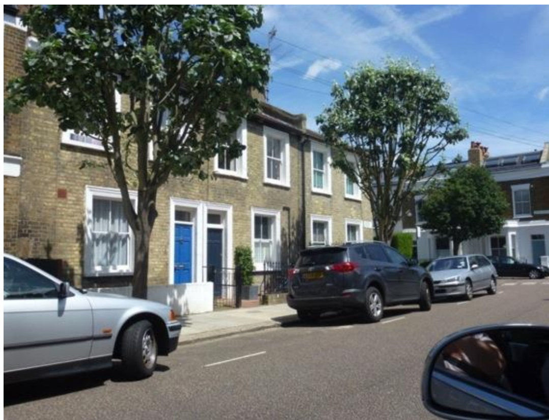
Two storey cottages in Furber Street – note the plaster mouldings around doorways and windows; timber sliding sashes and plain lights above solid six panelled timber doors. The neat simplicity and elegance of these mid-19 th Century cottages have been preserved and maintained.
