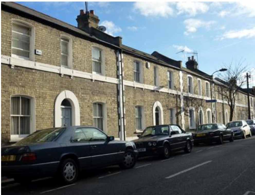
Cottages on the east side of Lamington Road.
