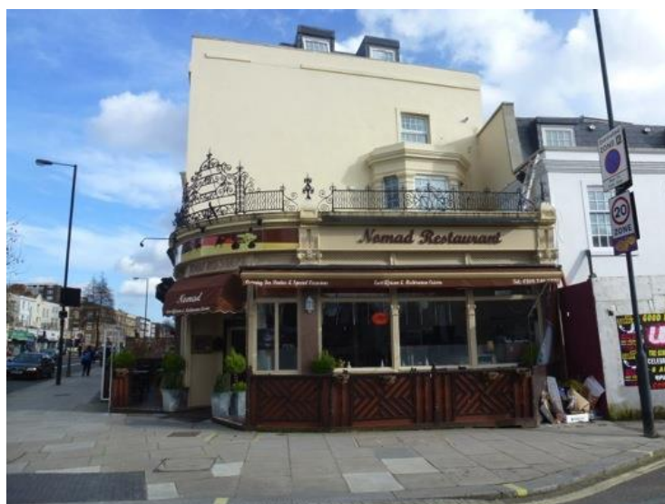
Now a restaurant, much of the character of the former Brackenbury Arms Public House remains.
