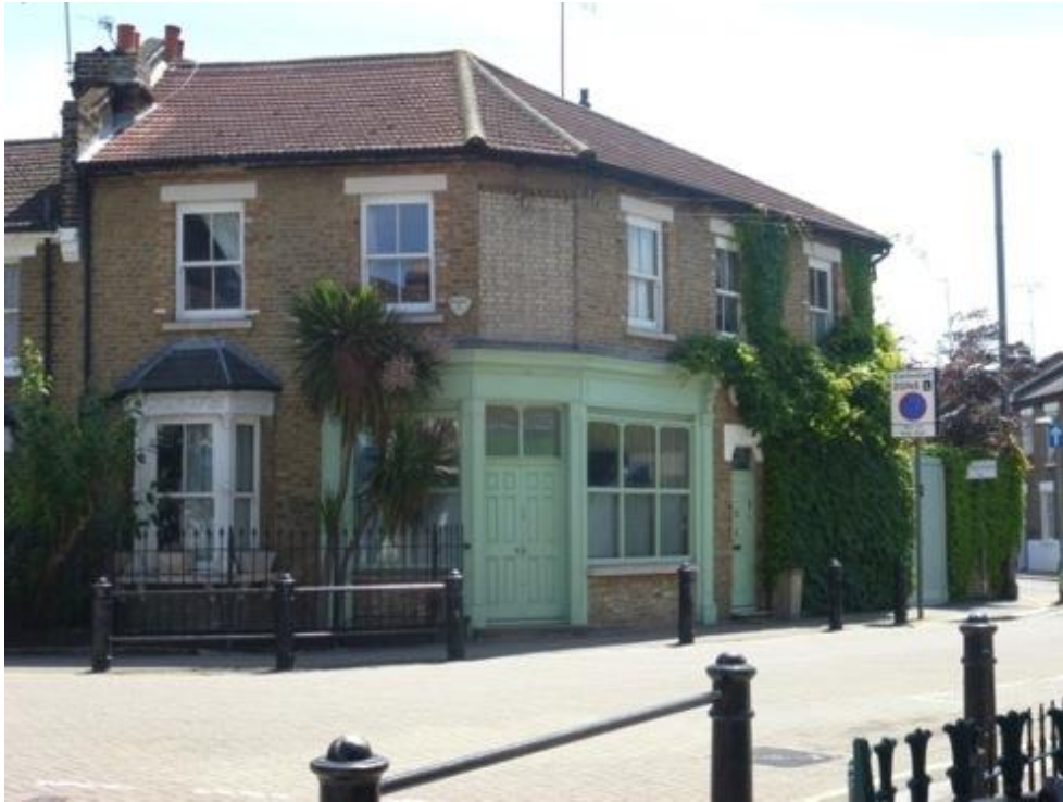
No. 51 Aldensley Road, once a corner shop.
