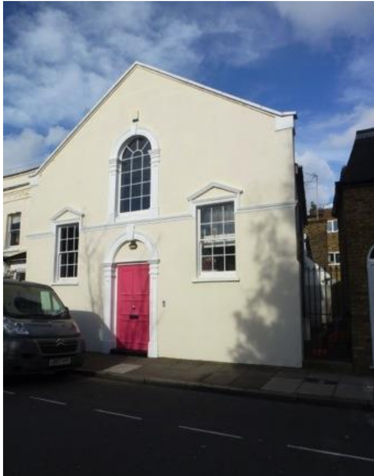
No. 40 Redmore Road, Emerson House – a former chapel building.
