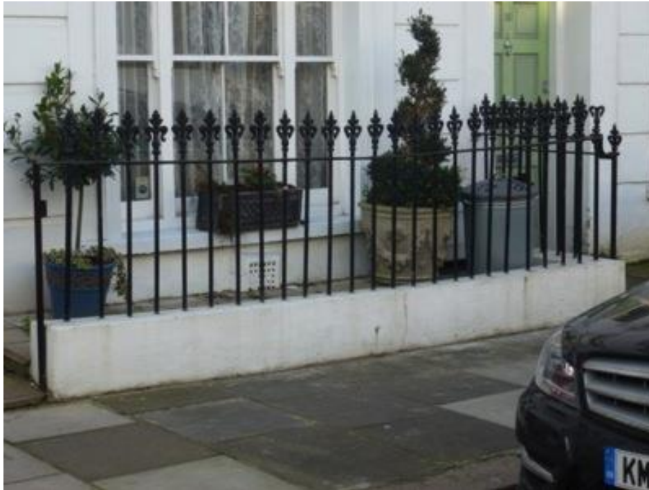
Detail of original railings in Raynham Road.
