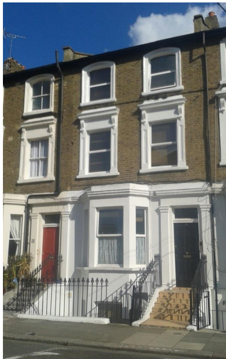
Stucco decoration is largely intact on the houses in Overstone Road.
