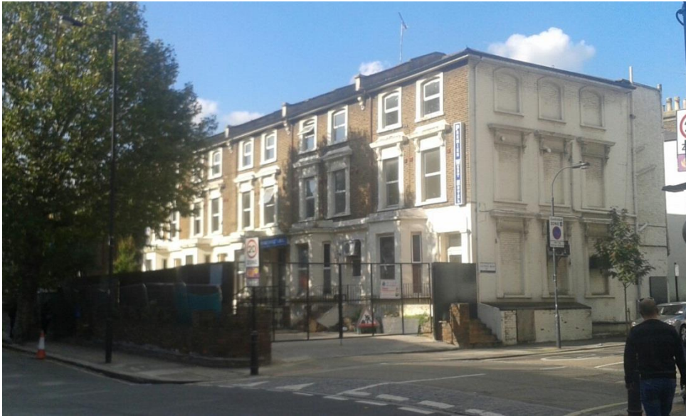
The Premier West Hotel prior to demolition.
