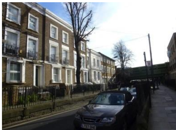
Properties on the west side of Cambridge Grove, showing the distinctive railings and the slope of the roadway as it sinks beneath the railway bridge in order to achieve headroom.
