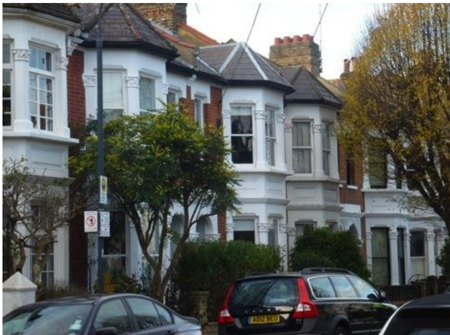
Properties on the west side of Iffley Road.
