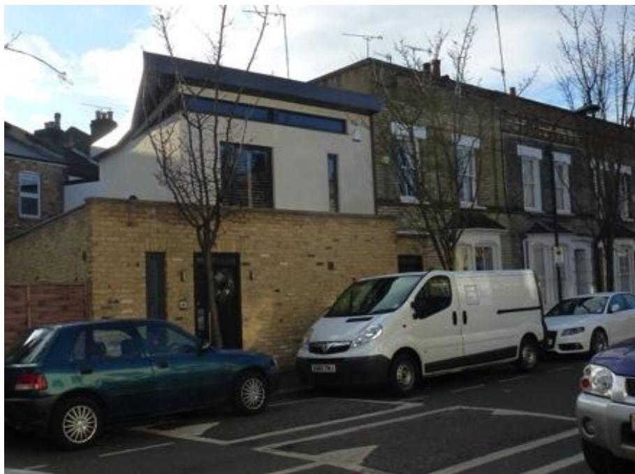
No. 29 Redmore Road – a successful modern intervention in the conservation area.
