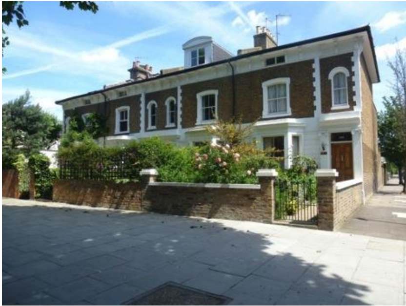
Nos. 134-140 Dalling Road – unfortunately the dormer extension, although well designed in itself, spoils the harmonious appearance of the roofline.
