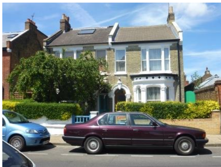
Nos. 203 and 205 Dalling Road.
