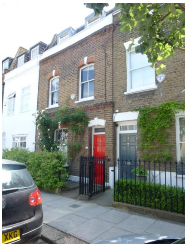
5-7 (odd) Furber Street (north side) showing the well-designed roof extensions that have been built on the entire group. The cottages on the north side retain their two storey character.
