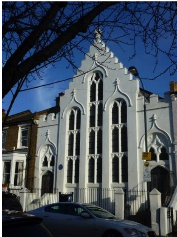
The western elevation of the former St. John's Hall.
