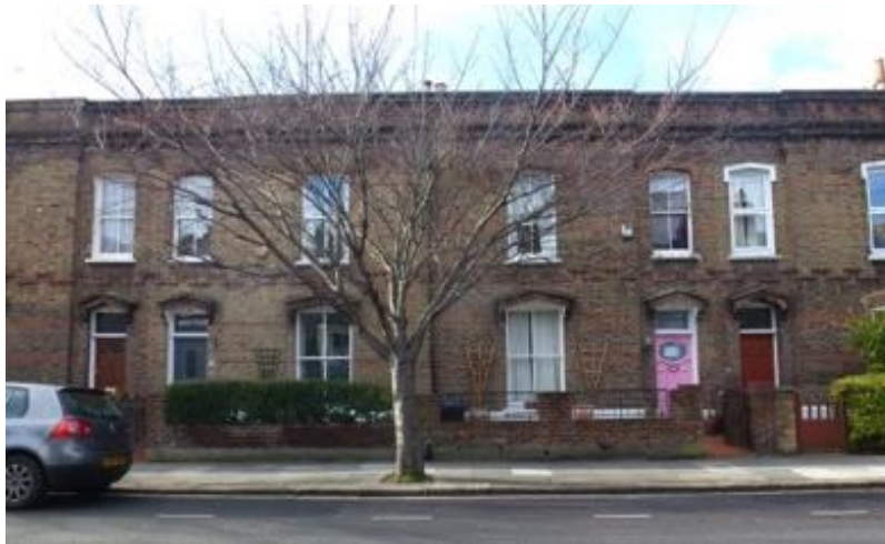
Nos. 19-21 Bradmore Park Road have shallow triangular brick pediments.
