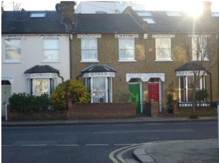
29-33 Aldensley Road, Cambridge House just visible behind.
