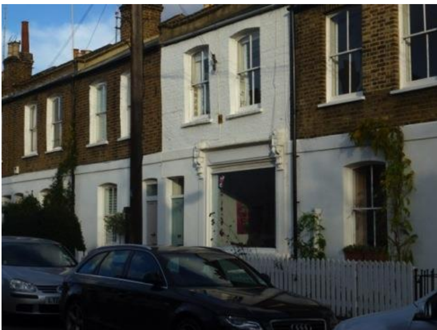
No. 75 Cardross Street – formerly a public house.
